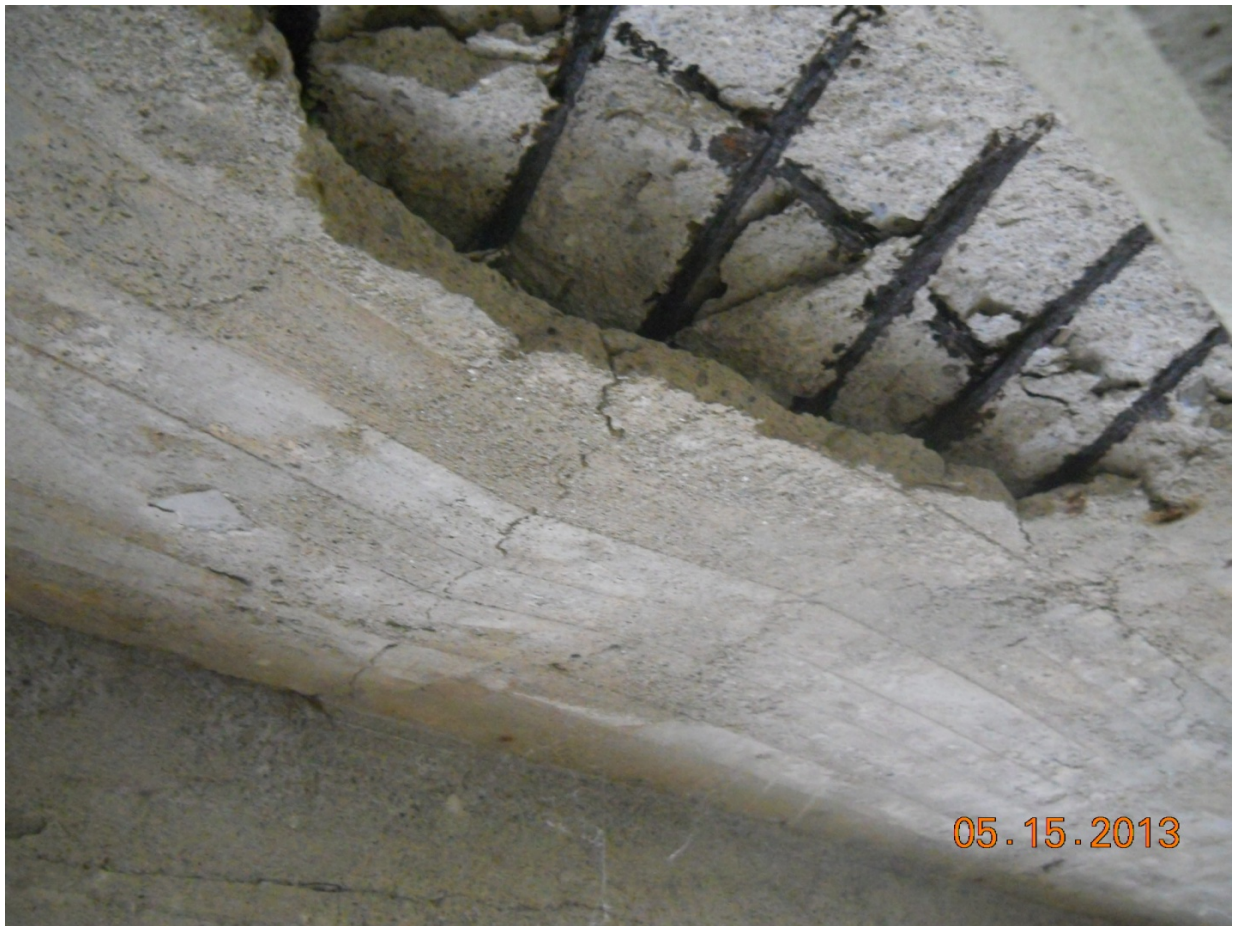
Deck Soffit Deterioration
